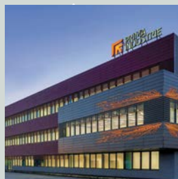
PRIMA INDUSTRIE HEADQUARTERS AND TECH CENTER Collegno (TO) - Italy
